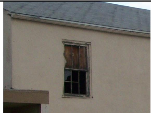
Figure 43: View looking southeast at a window on the former recreation building
