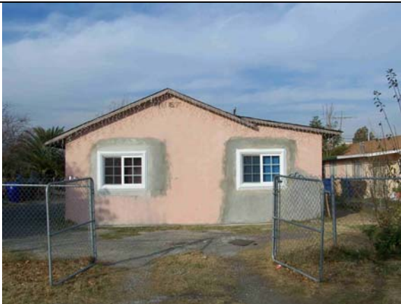
Figure 34: View looking north at the replaced windows of 8425, 27 Janet Avenue
