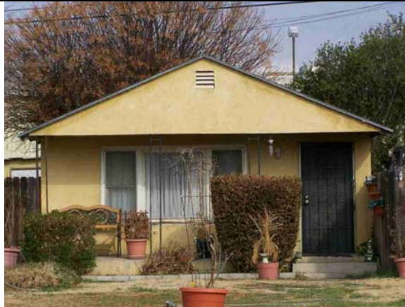
Figure 32: View looking north at the recessed entrance to 8395 Cypress Avenue
