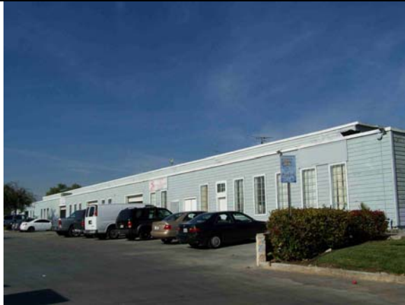
Figure 40: View looking northwest at the laundry facility
