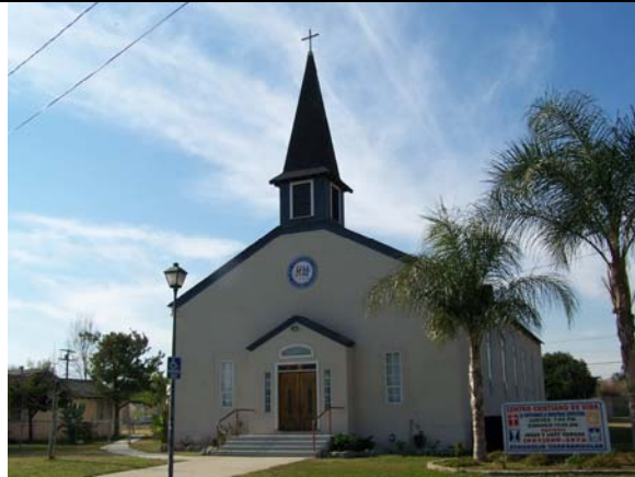
Figure 41: View looking southwest at the chapel
