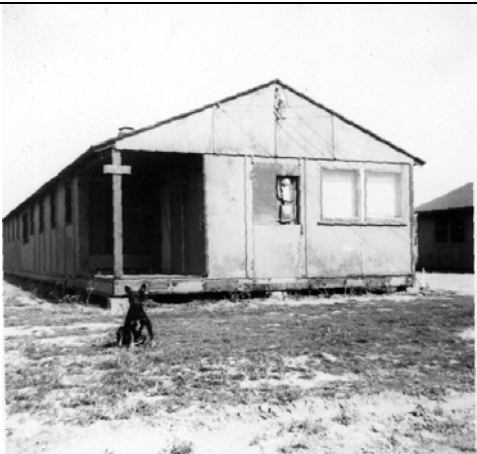
Figure 28: A 1948 view of a former officer's barracks in its original state (Frank Teurlay)
