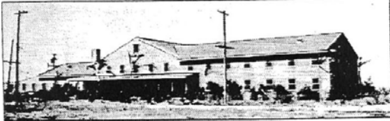
Figure 7: Circa 1947 view of the Service Club building (National Archives and Records Administration Pacific Region)
