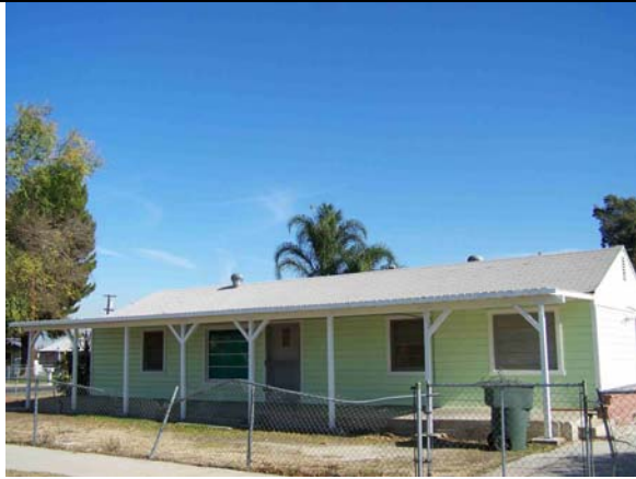
Figure 24: View looking northeast at 8022 Cypress Avenue
