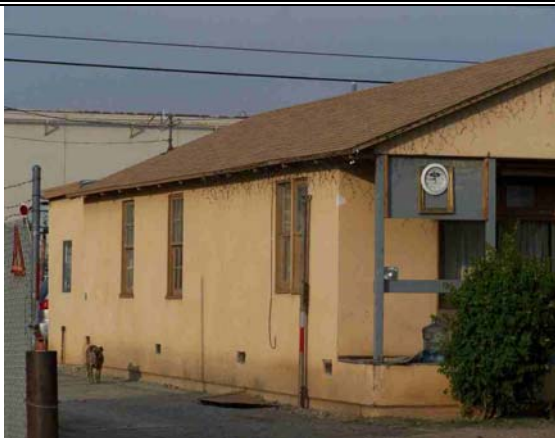
Figure 26: View looking northeast at the post-war era stucco cladding and fenestrations of 8553 Cypress Avenue
