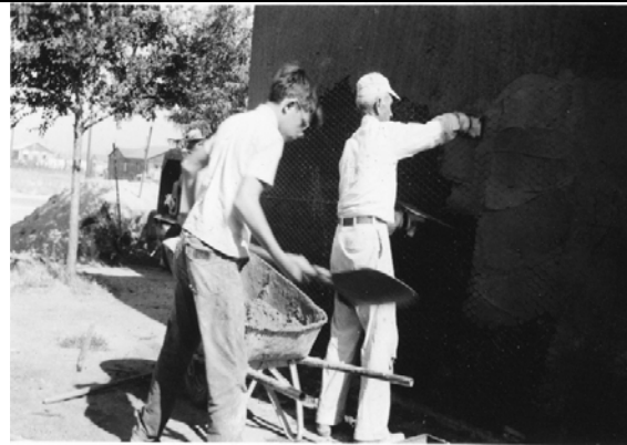
Figure 25: 1952 image of a plasterer applying stucco to a former barracks building (Frank Teurlay)
