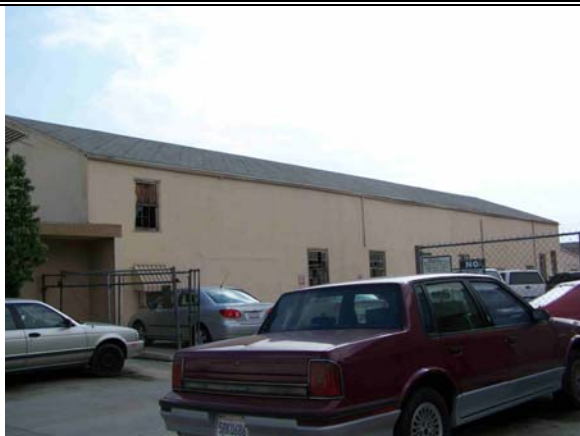
Figure 42: View looking southeast at the former recreation building at 7590 Cypress Avenue
