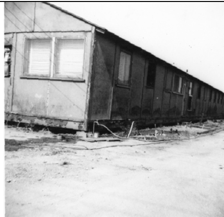
Figure 29: A 1948 view of a former officer's barracks in its original state (Frank Teurlay)
